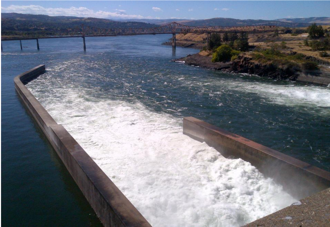
Spill attraction flow test for north fishladder. Results pending.
